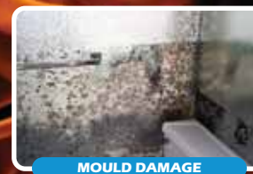
MOULD DAMAGE
